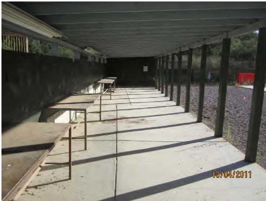
Photo 4 Interior of Covered Firing Area Photo taken facing South
