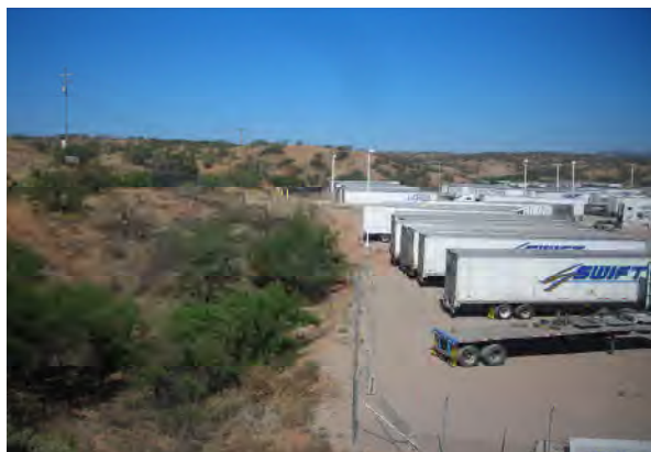
Photograph No. 7 Subject property (Looking West from Northeast corner where fence encroaches onto property)
