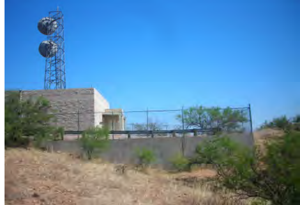
Photograph No. 10 AT&T Tower located on adjoining parcel enclosed by Subject Property
