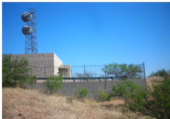
Photograph No. 10 AT&T Tower located on adjoining parcel enclosed by Subject Property
