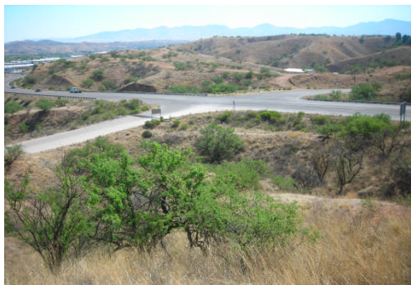
Photograph No. 9 Subject property (Looking Northeast at Mariposa Rd & Target Range Rd Intersection)
