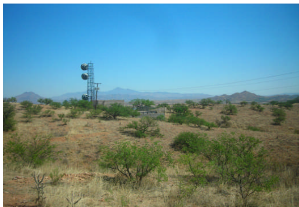
Photograph No. 11 AT&T Tower located on adjoining parcel enclosed by Subject Property
